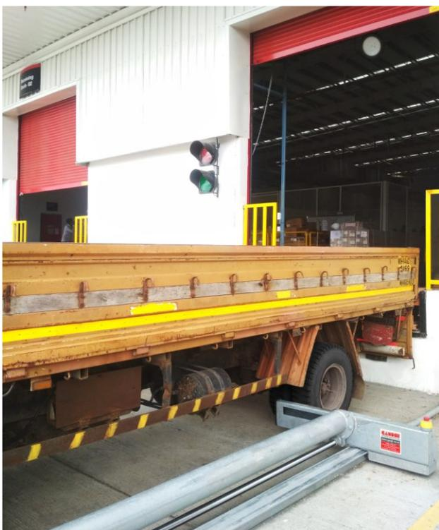
An integral sensor in the wheel block accurately determines the position of the rearmost wheel, where upon the wheel block is automatically extended and the wheel is restrained.
